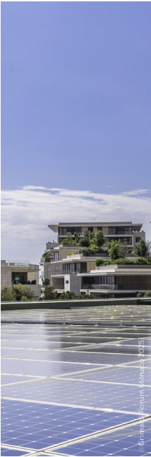
Photovoltaic panels set up on the roof of the GFM.
